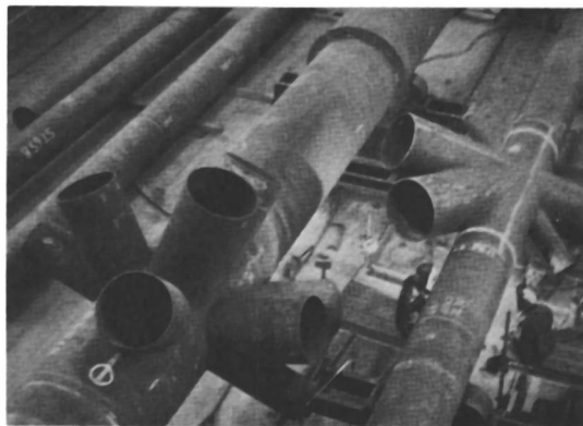
Figure 15. Off-shore platform node construction showing the complex welding assembly job requiring outstanding resistance to lamellar tearing in the electric-resistance-welded (ERW) steel pipe stock. Excellent through-thickness ductility is obtained by low sulfur plus REM treatment in the ladle, plunging a mischmetal canister.
