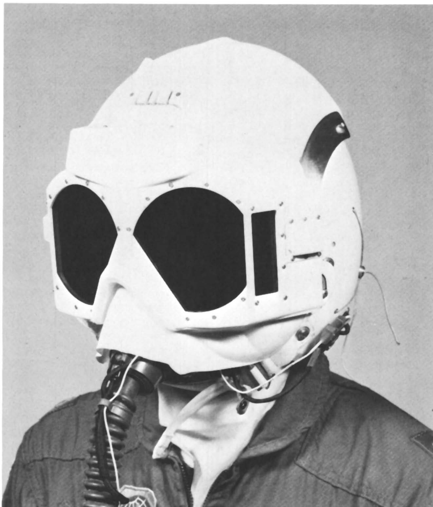
Figure 9. PLZT Thermal/Flash Protective Goggle developed by Sandia Laboratories for the U.S. Air Force
